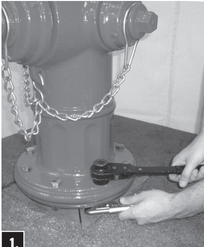
1. Loosen Nuts on Safety Flange Bolts.
