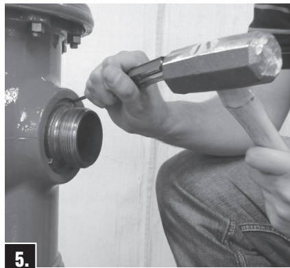
5. Remove Nozzle Cap and A-316 Nozzle Wrench. Place the Nozzle Lock (Part 143137), lengthwise in the slot formed by the Nozzle Drive Lugs and the Barrel Bore. Drive the Nozzle Lock in place by striking the Nozzle Lock Installation Tool (Part 143132) several times with a heavy brass hammer.
