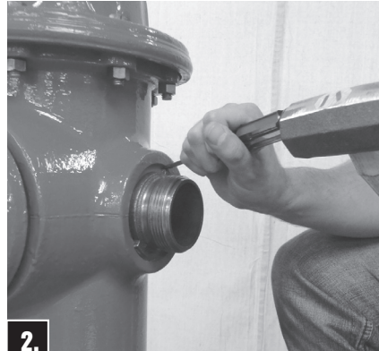
2. Remove stainless steel Nozzle Lock by driving it out with a pointed tool and hammer.
