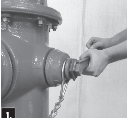
1. Remove Nozzle Cap.
